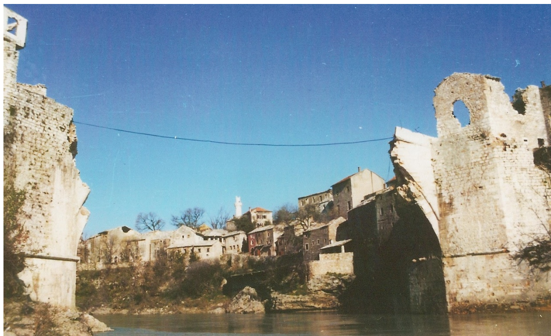
Sl. 1. Srušeni Stari most
